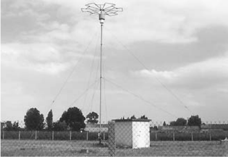
Figure 4-36. NDB nondirectional beacon. (Source: FAA)
